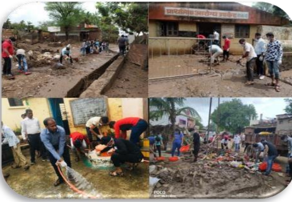
Flood Area Cleaning
